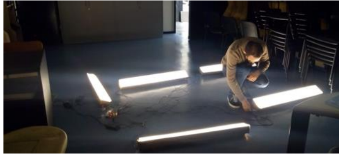
Fig. 3. Picture of the Dynamic Lighting System installation inside the laboratory
